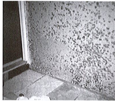
Fungus and mold spread in wall
