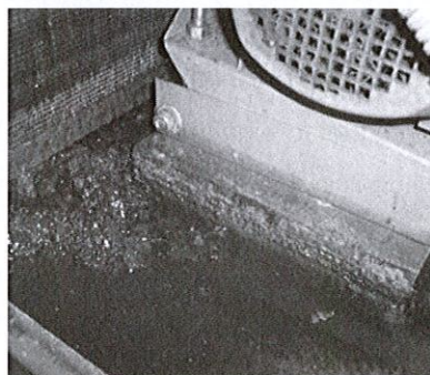
Improper maintenance of HVAC system
